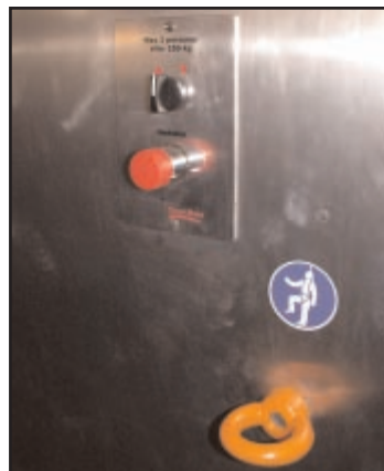
Control Panel and anchor eye attachment point for operator's safety harness when evacuating cabin in an emergency situation.
