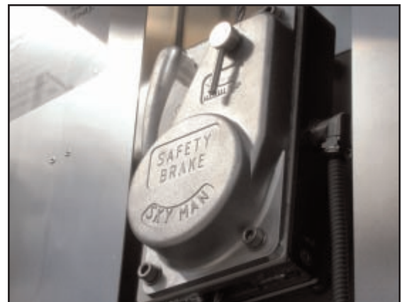
Overspeed safety brake inside cage. Pulling handle provides emergency descent at controlled speed in case of power failure.
