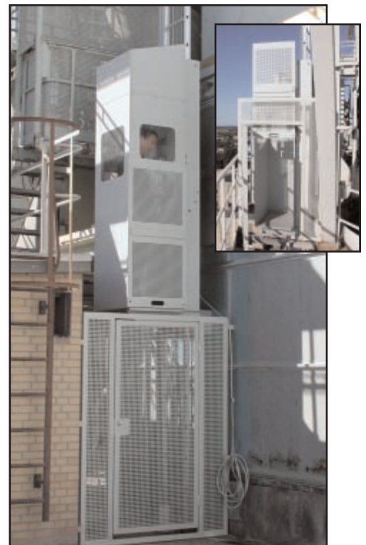
Example of cage arriving at base of tower into security enclosure (by others).
